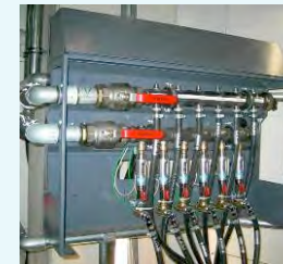
Chill water console
